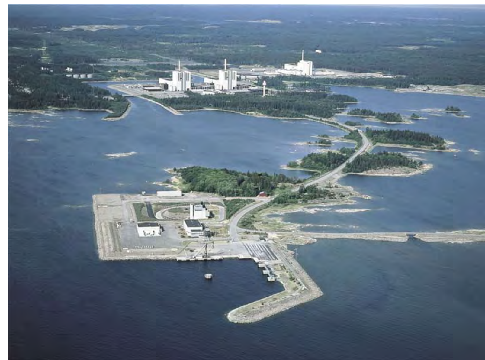
The SFR in Sweden manages L & ILW in bedrock caverns 60 metres below the Baltic Sea.
